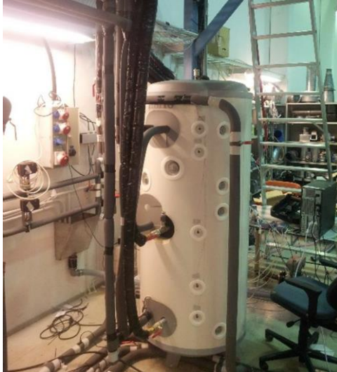
Figure 20. One of the hot water tanks, and schematic of the storage tank connections.
